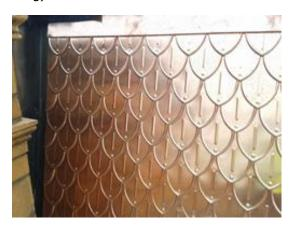
VMZINC Ornaments has a tradition of zinc and copper ornamental work for roofs which date from the first half of the  $19^{\text{th}}$  century. Its extensive list of commissions is now showing a steadily increasing number in the UK. Such rare belief in the retention of key metalworking skills enables historic buildings to be restored and elements of the roof retained as key building features.
