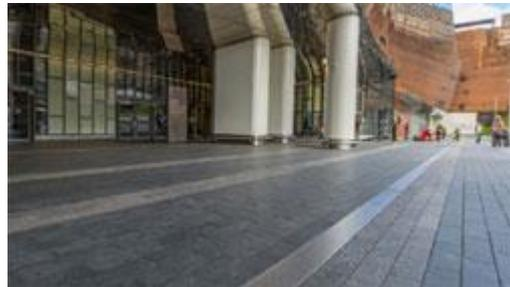
ACO Building Drainage designed a bespoke radial channel solution with 6mm uniformed joints which matched the channel covers provided by ACO Water Management. The team also designed an outlet for the channels, enabling them to deal with the deep slab design and technical practicalities of the site.
