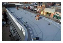
Surface preparation and conditioning was carried out to provide a suitable substrate onto which the Caltech UV BUR system could be applied.
