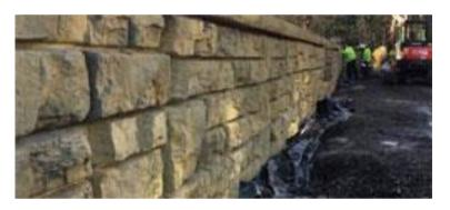
The final design cover over 600 metres of flood defences by means of a combination of earthen raised bund through agricultural land, plus a 1.5-metre-high modular block wall, complete with gates and demountable barriers, where the line comes closer to a domestic property.
