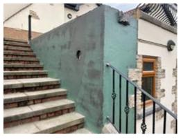
Where different types of construction meet, there is always potential for movement. Koster NB 4000 would provide a long lasting, flexible approach in providing security for difficult junctions and the event of movement. Koster NB 4000 is an elastic, crack bridging, bitumen free, polymer modified, mineral hybrid coating suitable for external waterproofing application. Being UV stable, and not weather dependant, an ideal remedial solution for this project.
