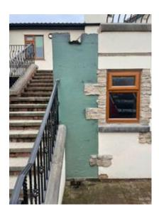
At the time of the construction, the podium deck had been waterproofed, however detailing to the parapet and surrounding wall was poor. The parapet and external wall itself had been left completely unprotected and vulnerable. Over time, water inevitably ingressed into the structure.
