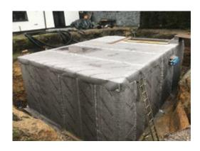
When designing a robust waterproofing approach, attention to detail is critical. Working in collaboration with the ground works team, Dryside Ltd were able to ensure all construction joints and service entry points, were sealed to a high standard.
