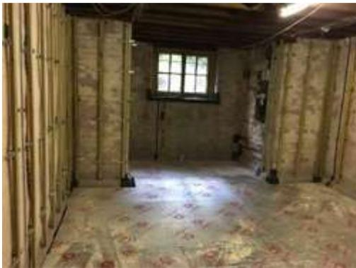
Contractor Timberwise was called upon to investigate the damp issues and to suggest remedial options which would incorporate BS 8102:2009. All basements should be constructed (or retrofitted) to cope with groundwater levels up to the full retained height of the basement. Structural waterproofing preserves the integrity of a structure whilst ensuring the usefulness of the building for present and future use.
