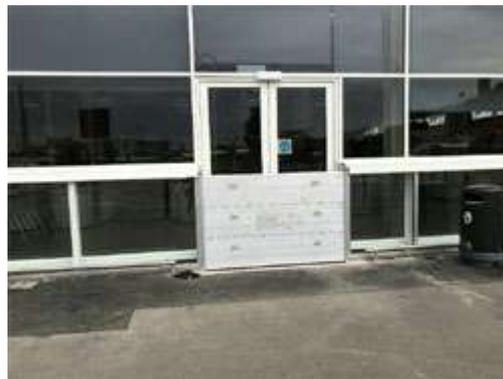
The Flood Company was called in to survey the site and devise flood prevention measures that could be retro-fitted to the building. The Buffalo Panel System was chosen as a way of creating an exterior flood proof seal that would match the appearance of the supermarket. The Flood Company also installed Buffalo Glass, which provides a visually appealing barrier for use in public areas, as well as a Buffalo HD Barrier System around doors and loading bays.
