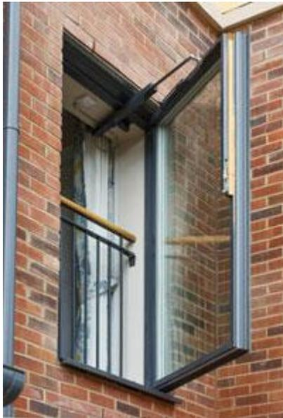
A total of 16 GEZE [RWA 110 NT](#) window actuators were installed in pairs throughout the corridors of the three-storey building which is managed by Rapport Housing & Care. These incorporate an electric spindle drive which is coupled with a mechanical locking mechanism.
