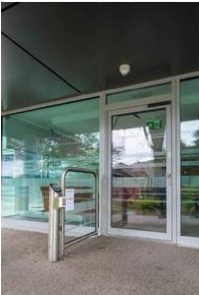
Set alongside it, is a [Slimdrive EMD-f](#) automatic swing door - one of 15 fitted in the redevelopment - which operates a door that has been added for increased accessibility. The electro-mechanical swing door mechanism makes it extremely versatile, providing easy access for those with mobility issues. Assisted opening can be initiated using the operating button with guaranteed constant opening and closing speed.
