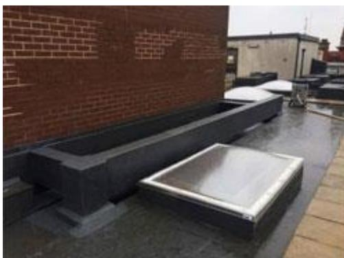
Contractors had to clean the roof prior to the application of Kemper System's Kemperol® V210. The lack of drainage meant any power washing created more ponding on the roof. Therefore, contractors used a vacuum wash and dry system that automatically extracted the waste water and pumped it directly down the drainage outlets.
