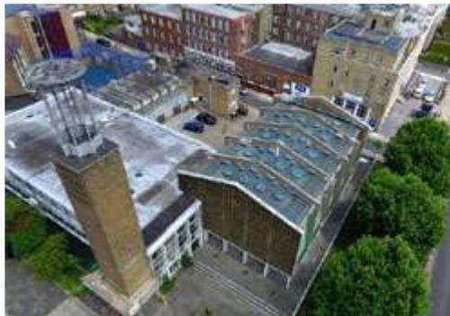
For many years, financial challenges meant the church had to carry out temporary repairs, which included a timber structure built over the entire roof area, and a felted covering on top of the original roof surface.
