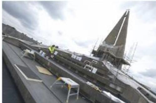
The technical team at Kemper System also devised a series of drainage channels to address the volume of standing water on the roof, whereby excess water would be caught and drained off the building.
